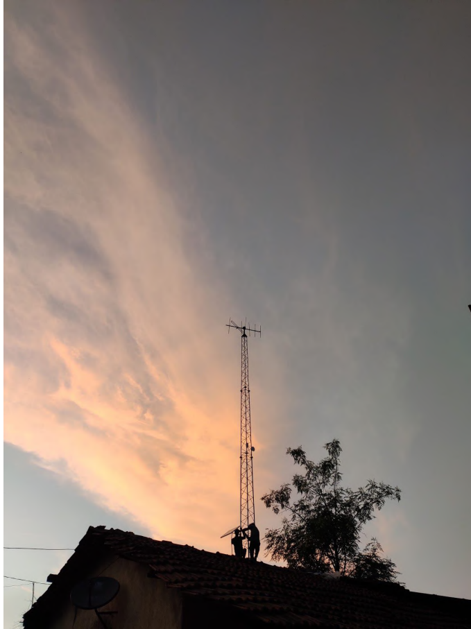
Figure 14: Deployment on the tower at Ramkhind.
